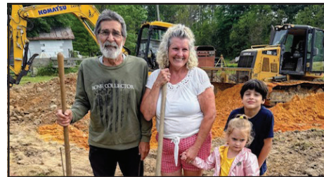
The groundbreaking for the new home was held April 18, 2026, and approximately thirty loads of dirt was donated for the pad and foundation.
